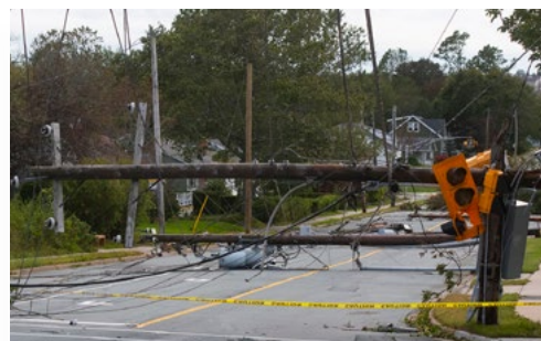
Downed power lines in Dartmouth, Nova Scotia. (photo: SaltWire/Ryan Taplin)
