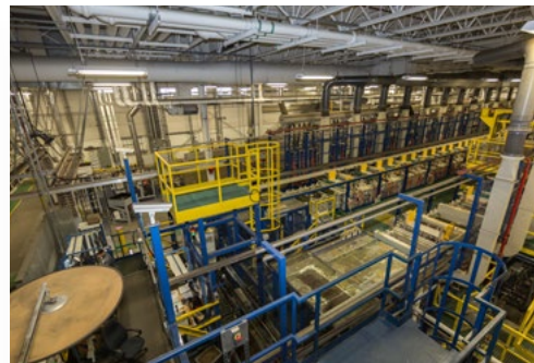
The Mint has committed to making its Winnipeg facility carbon-neutral by 2030.
