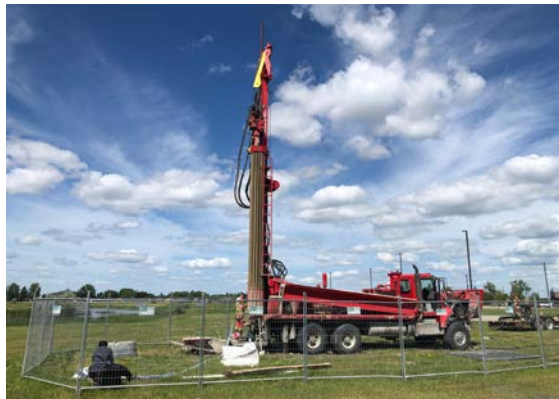
Geothermal pipe installation in Winnipeg
